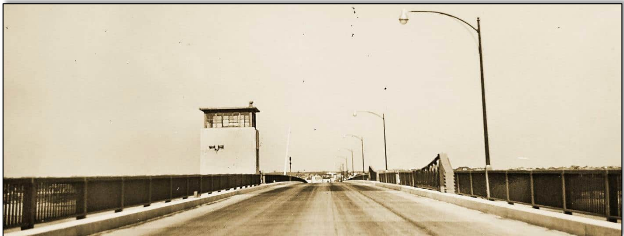
Recently completed bridge, view of deck, control tower and draw in down position, looking north, August 31, 1950. Photo from NH Highway Department bridge inventory card.
