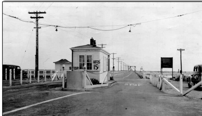
Toll booth at Seabrook end of bridge. The overhead timber frame supporting the lifting cables for the bascule draw span is visible in the distance. No plans or photos of the draw were located. This photo and one below taken July 1, 1940 by NHHD during inventory of the state's bridge conducted just prior to World War II (Bridge inventory card, Hampton 300/043).
