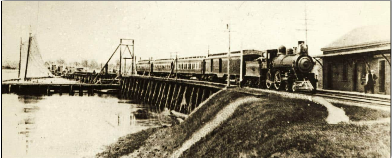
Eastern Railroad train crossing the Piscataqua River bridge from Portsmouth and arriving at the Kittery Depot. Behind the train is an upright shear-leg or "shear-pole" framework that supports the swing draw when it is opened. Another shear pole swing draw was located at the west end of the bridge between Noble's Island and the shore. Courtesy of Portsmouth Athenaeum.
