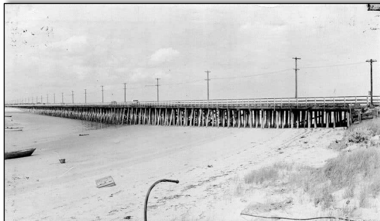
The trestle was carried on an estimated 870 timber bents. A typical bent as shown below consists of wood pilings joined with timber bracing. A heavy timber cap rests on the piles and carries the deck stringers, to which the decking, curbs and railings are attached. At each end of the bents were "batter piles" that were driven at an angle and bolted to the bent to brace against the forces of ice, boats and flotsam driven against the trestle by wind and tides.
