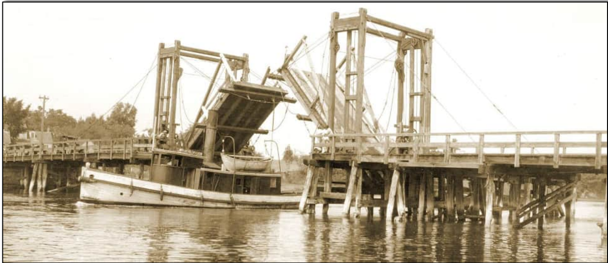
Stratham Bridge over Squamscott River, photo ca. 1920, showing the double-leaf, cable-lift bascule draw span built 1884. Courtesy Stratham Historical Society.
