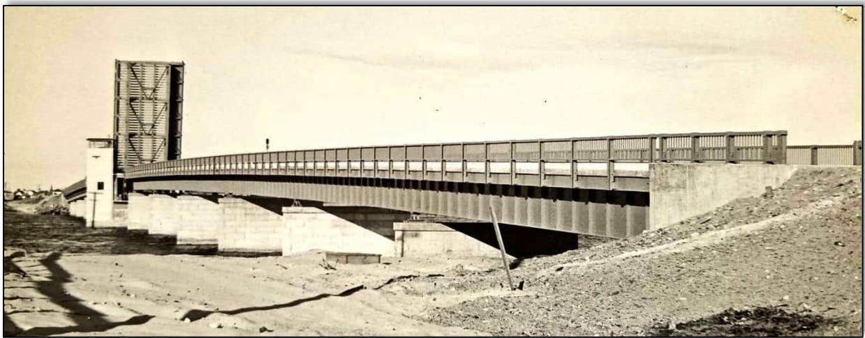
Recently completed bridge with draw span raised, west side, looking northeast, August 31, 1950. Mile Long Bridge remains standing out of view at left, evidenced by shadows. Photo from NH Highway Department bridge inventory card.
