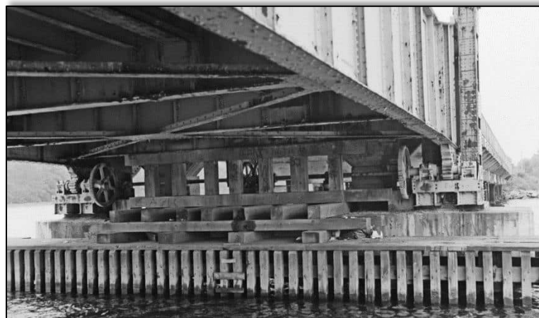
Below: Underside of lift span, showing lift gear machinery.
