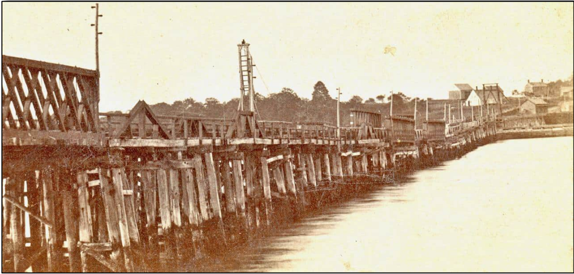
Portsmouth Bridge was a wood pile trestle highway bridge that stretched 1600 feet across the Piscataqua from Portsmouth to Kittery. Extreme currents, tidal range and depth of water made the bridge a monumental undertaking few thought feasible. This photo, ca. 1885, courtesy of Portsmouth Athenaeum, shows the downstream side of the Eastern Railroad trestle, built 1842, immediately alongside the Portsmouth Bridge.
