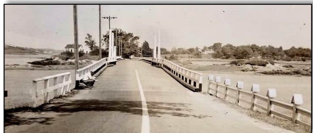
Below: West approach to middle trestle of the bridge taken July 3, 1940 by NHHD bridge inspector Wendell H. Piper.
