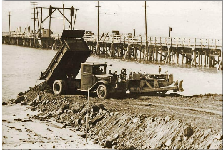
Construction of gravel filled approach causeways for the Underwood Bridge on the seaward side of the Mile Long Bridge, visible in background, in the fall of 1947 (Courtesy Lane Memorial Library).
