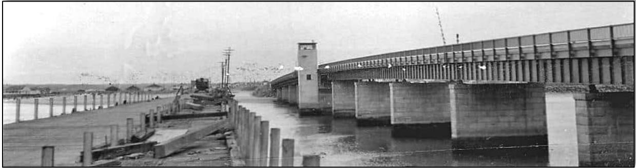
Underwood Bridge completed, 1950, with Mile Long Bridge awaiting demolition. Photo courtesy of Lane Memorial Library.
