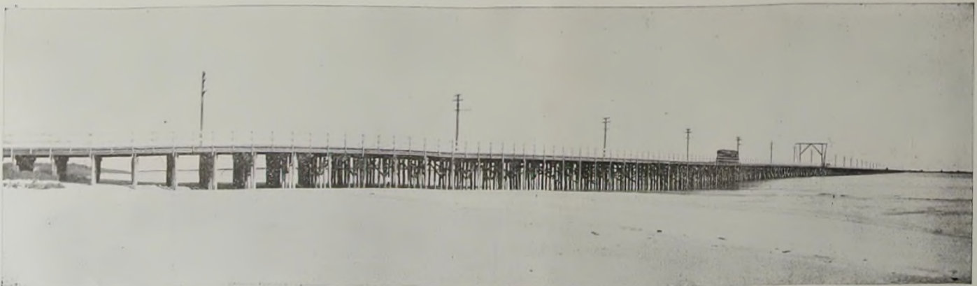
An Unusual View of the Great Hampton River Bridge
