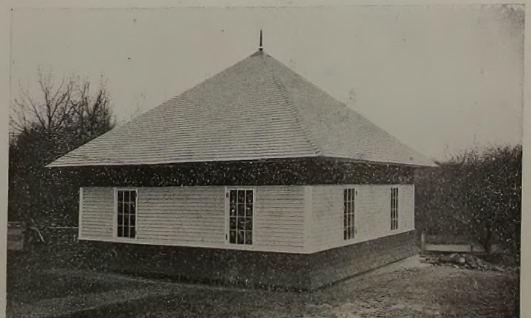
Pumping Station of Hampton Water Works
