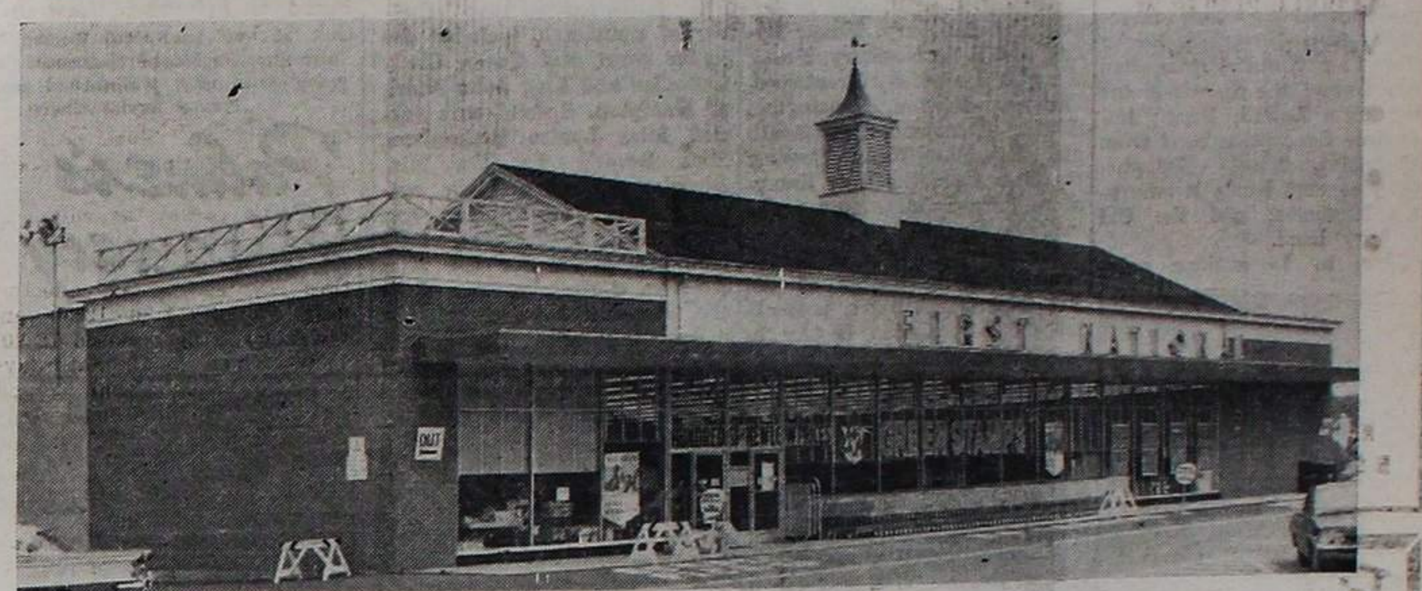
LAFAYETTE ROAD - ADJACENT TO LAMIE'S TAVERN
