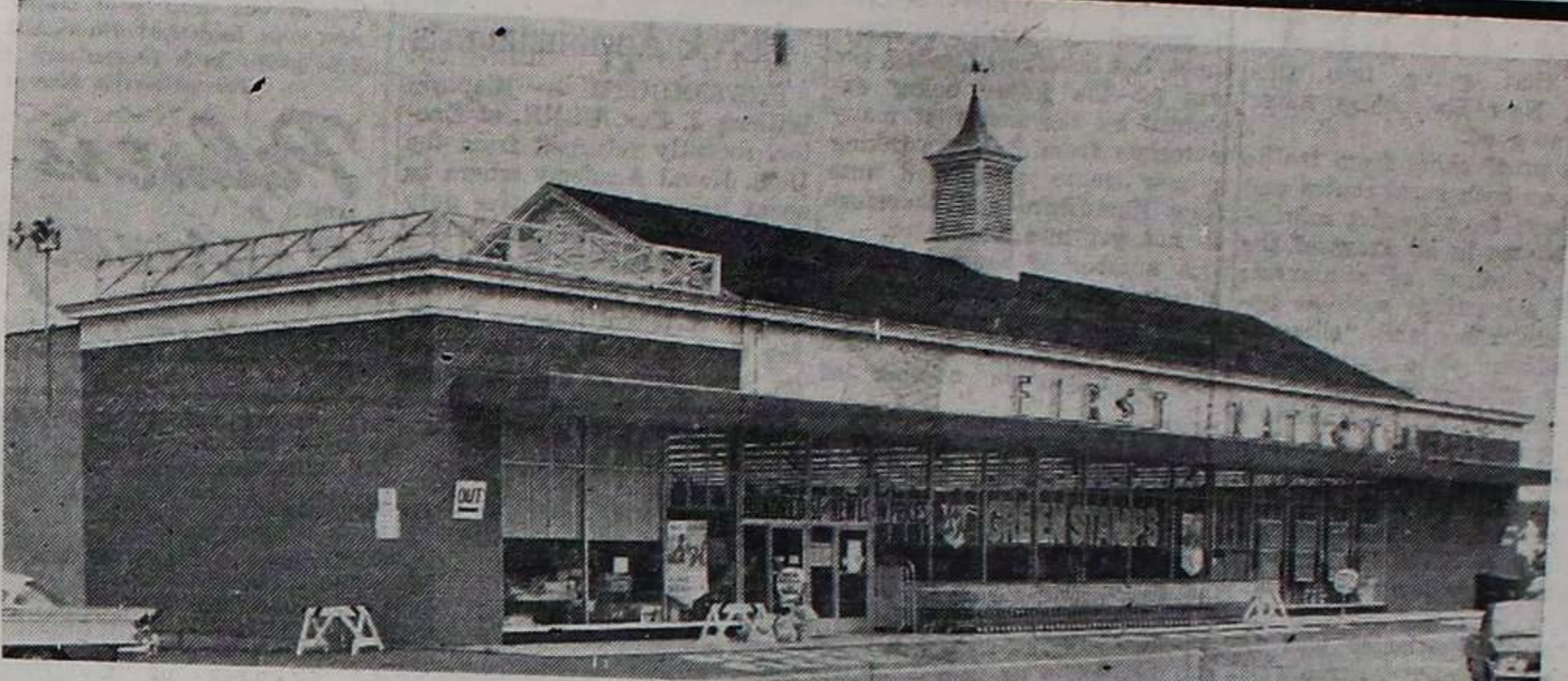
LAFAYETTE ROAD — ADJACENT TO LAMIE'S TAVERN
