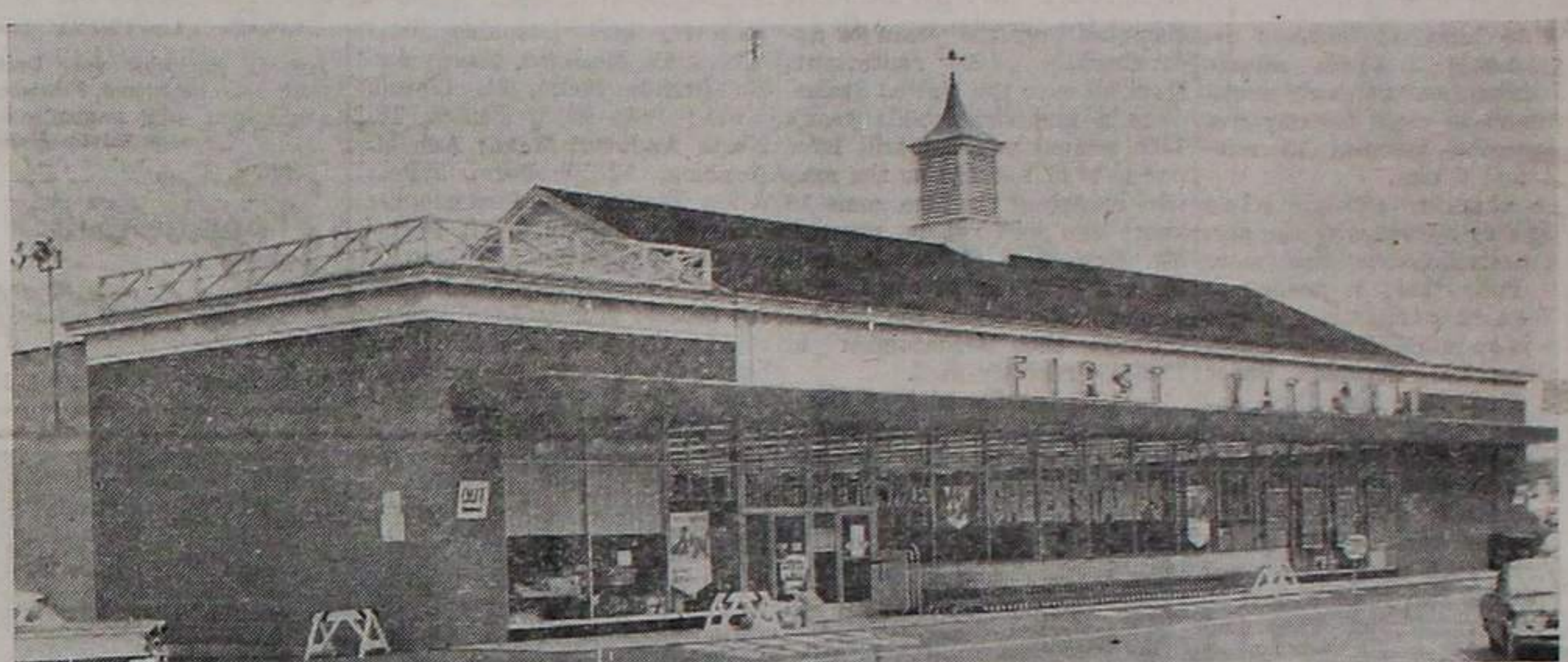
LAFAYETTE ROAD - ADJACENT TO LAMIE'S TAVERN
