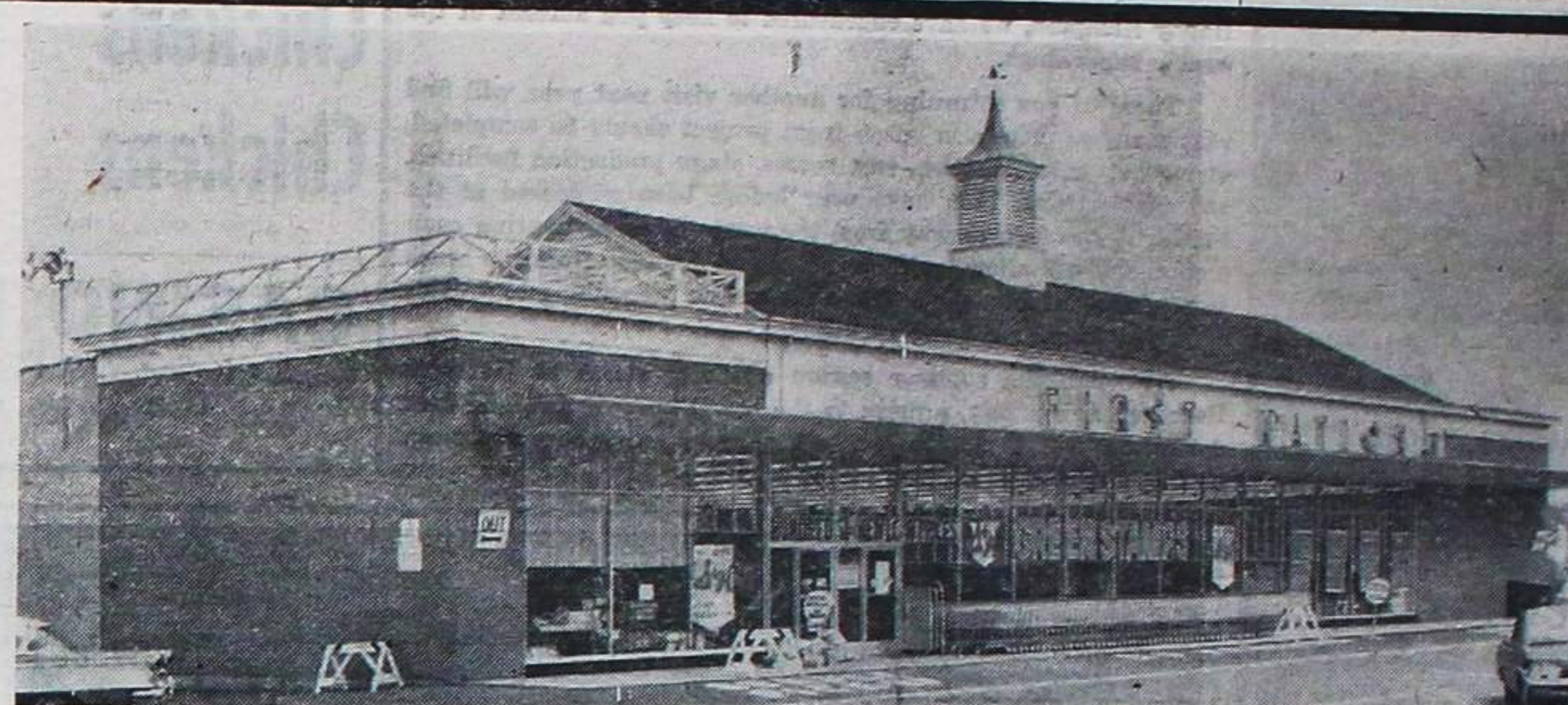
LAFAYETTE ROAD — ADJACENT TO LAMIE'S TAVERN
