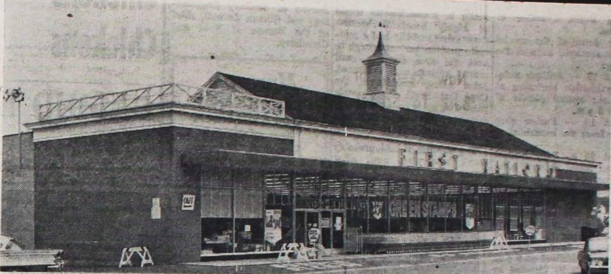
LAFAYETTE ROAD — ADJACENT TO LAMIE'S TAVERN
