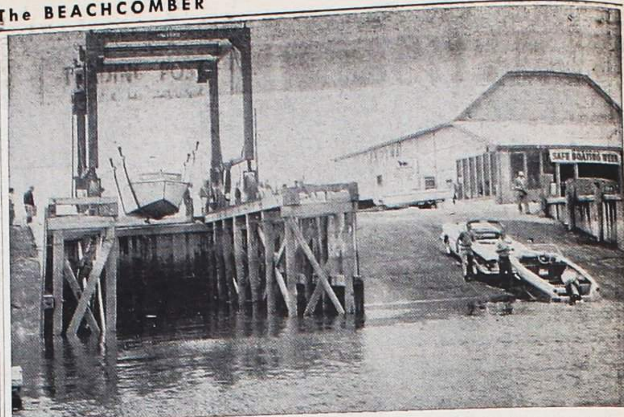
HAMPTON BEACH MARINA now provides complete launching facilities for boats of all sizes. Holly Hoist, at left, has a 20-ton lift capacity and launching ramps, at right, provide for launching of two smaller boats simultaneously. —Staff Photo
