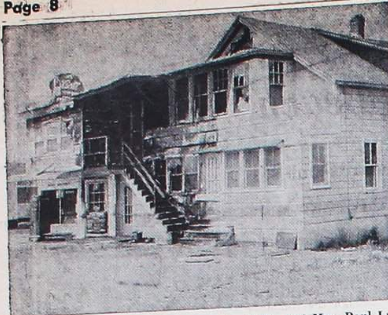
A MAJOR FIRE gutted the property of Mr. and Mrs. Paul LaRochelle, 39 King's highway, North Beach, Friday evening.
