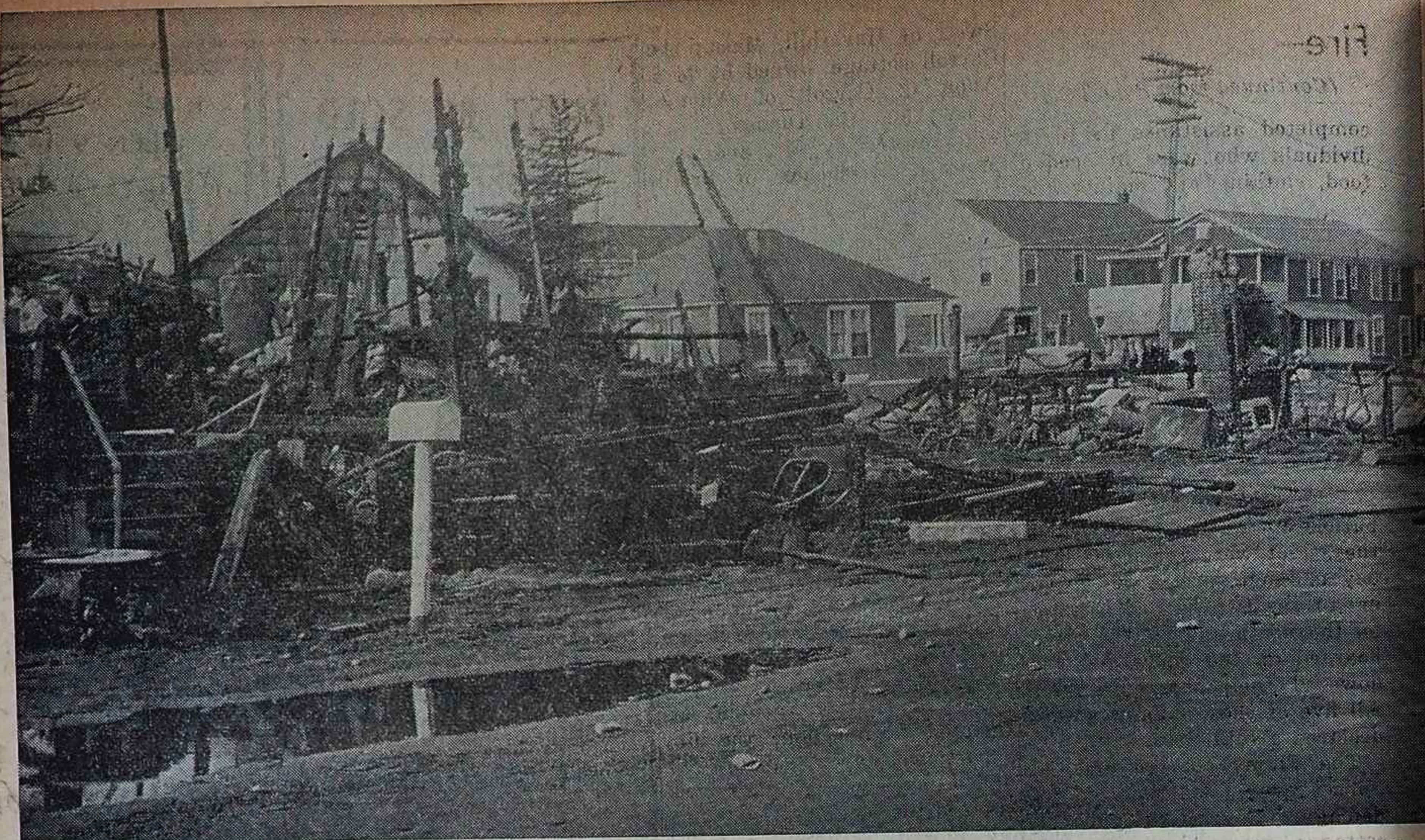
H STREET SUNDAY MORNING—Two rooming houses on the south side of H street were leveled in the conflagration Saturday night that roared through three other cottages, leaving only shells, and caused damage to two motels, including the Pigmy, left background. In the foreground are the ruins of the Roberta, left, and the Fireside as they looked after the sun came up Sunday morning. —Staff Photo
