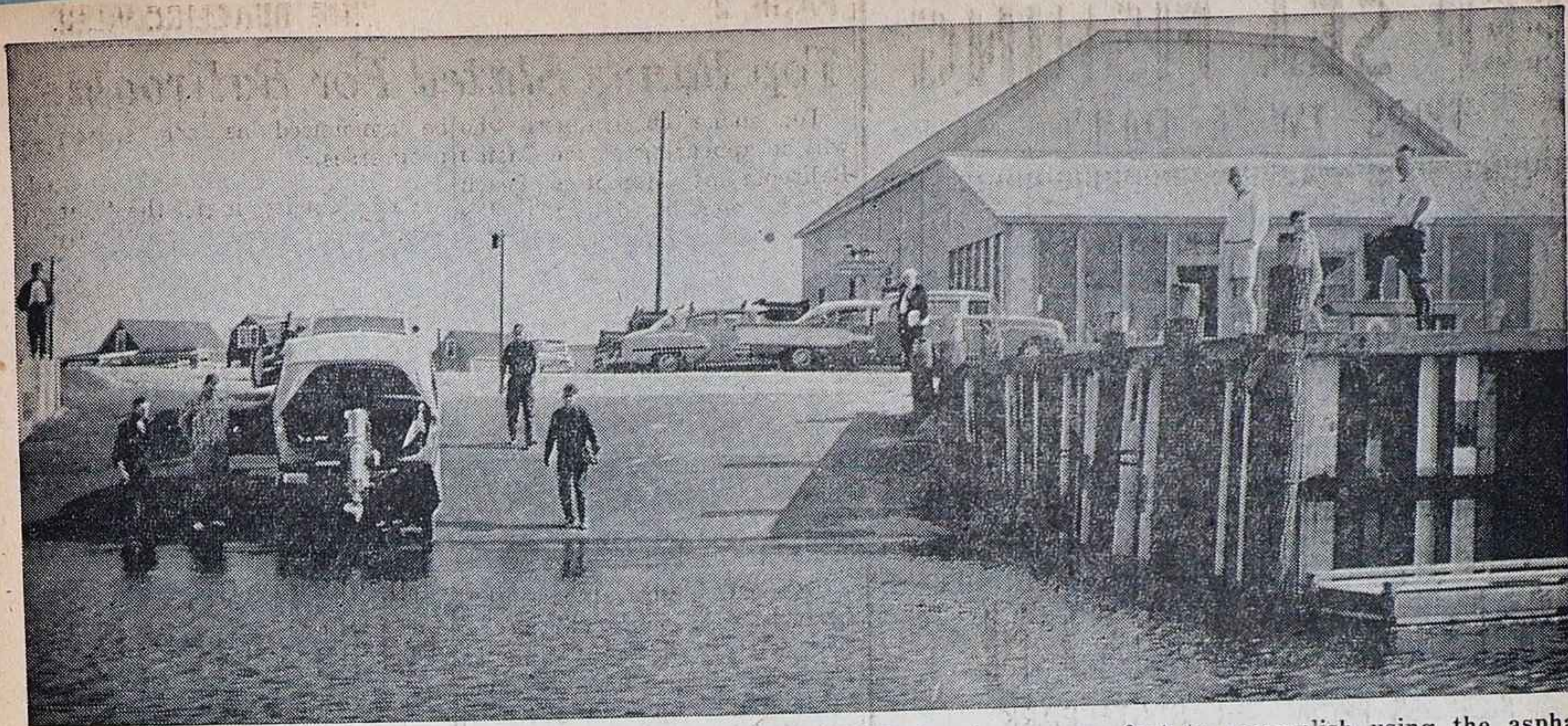
LAUNCHING A BOAT at the new facilities at the Hampton Beach Marina is an easy feat to accomplish using the asphalt ramp which is wide enough for as many as four boat trailers at one time. Usable at any tide level, the ramp went into service last week. Permanent and transient docking facilities are now available in the new Smith and Gilmore marina.
