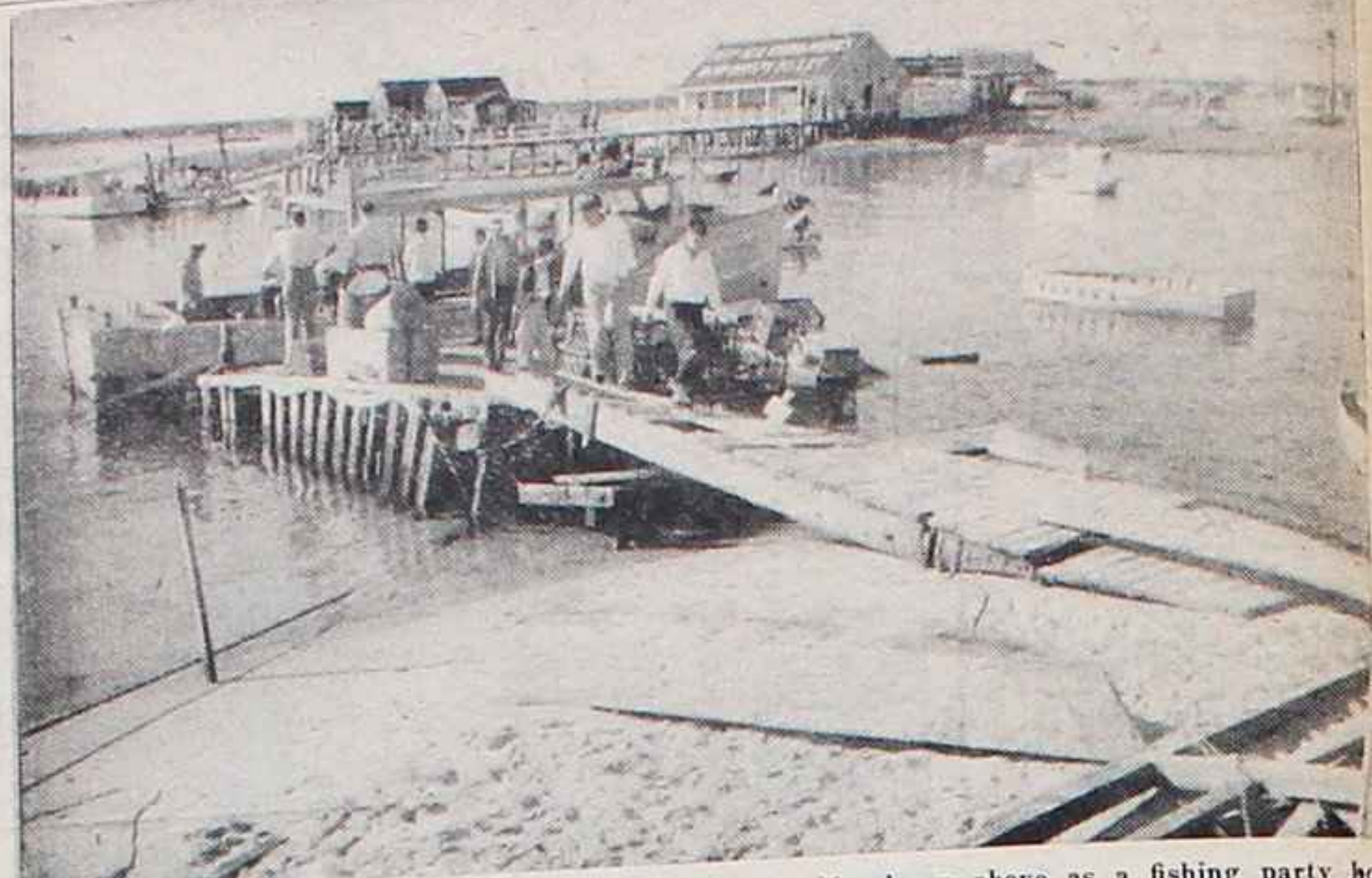
UNSAFE CONDITION of the state pier in Hampton Harbor is shown above as a fishing party boat attempts to land its passengers. Party and lobster boat operators have had to patch up the float as best they could in order to accommodate the hundreds of persons using the harbor facility every week.
