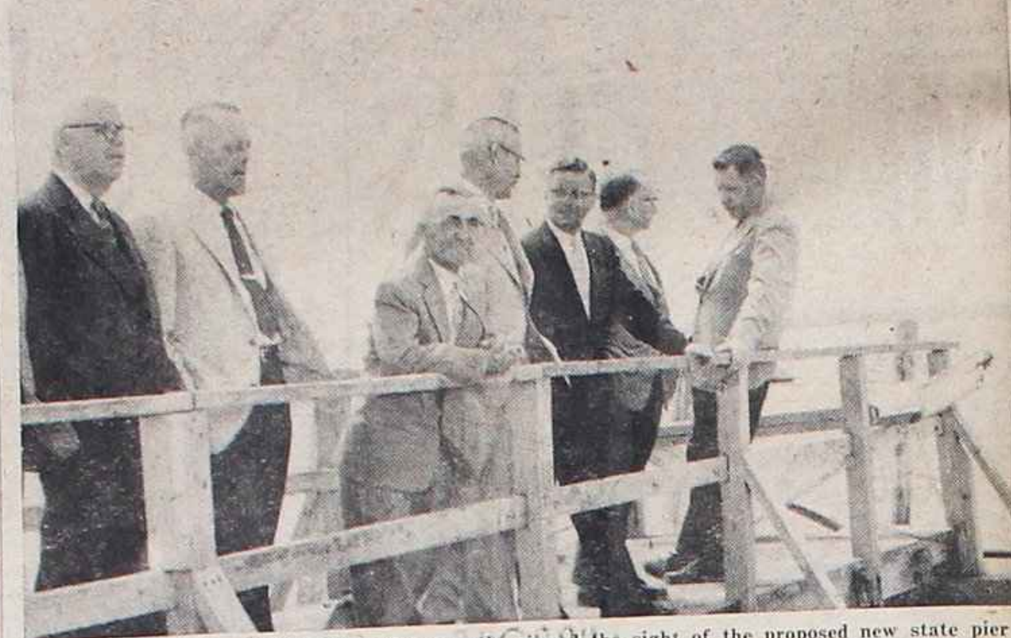
TOWN, BEACH AND STATE OFFICIALS recently viewed the sight of the proposed new state pier at Hampton Harbor to replace the present structure badly damaged by the elements. Forestry and Recreation department heads indicated that construction of the new pier hinges on legislative approval of funds.
