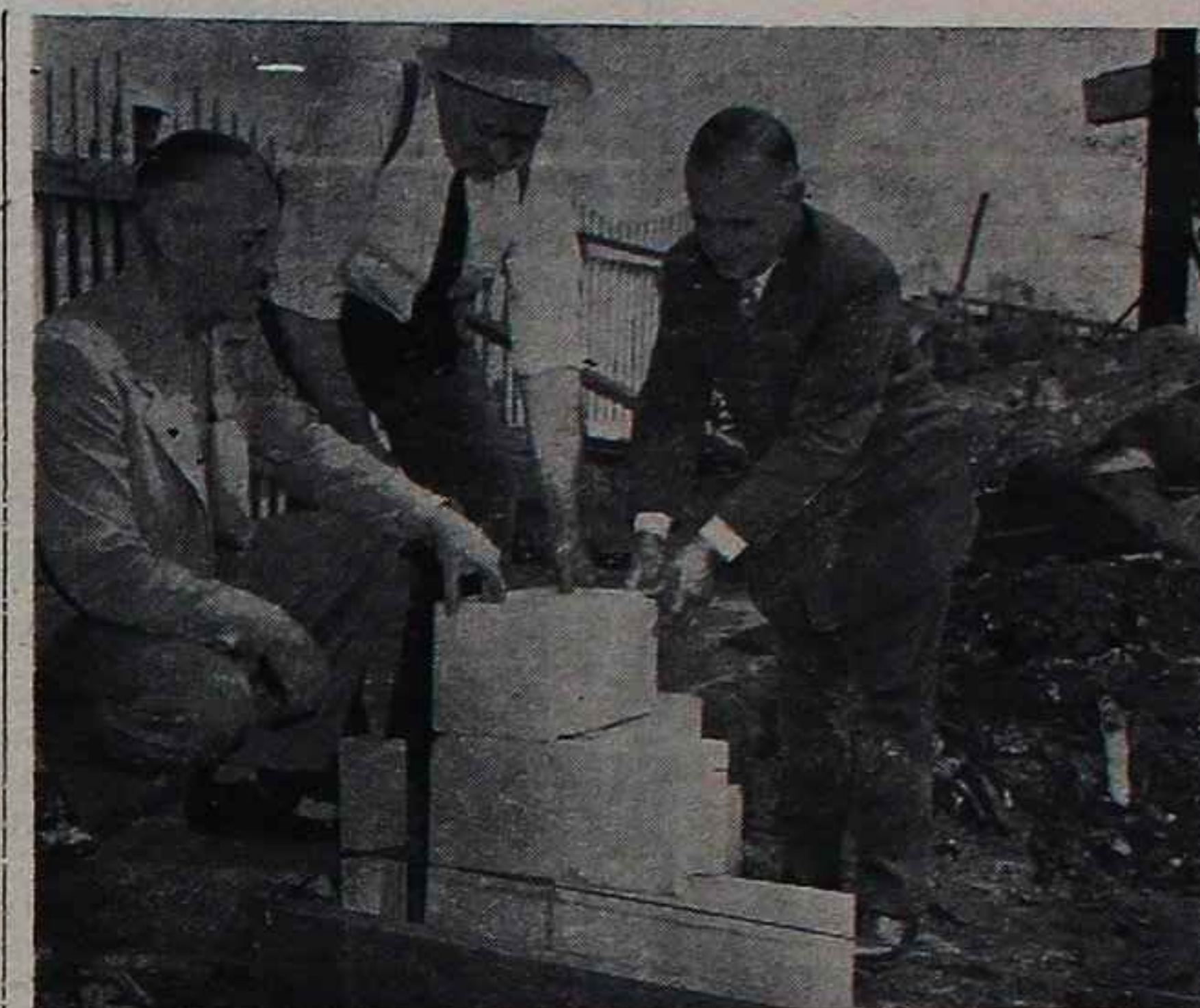
DEDICATION CEREMONY for the new modern business block to be built on the southerly corner of C street and Ocean Boulevard was presided over by Secretary Charles F. Butler of the Chamber of Commerce, left, Mr. Edwin L. Batchelder of the Hampton Beach Improvement company, center, and President Ray L. Goding of the Chamber of Commerce. Present plans call for work to be started on the new building next Monday. Photo by Marston
