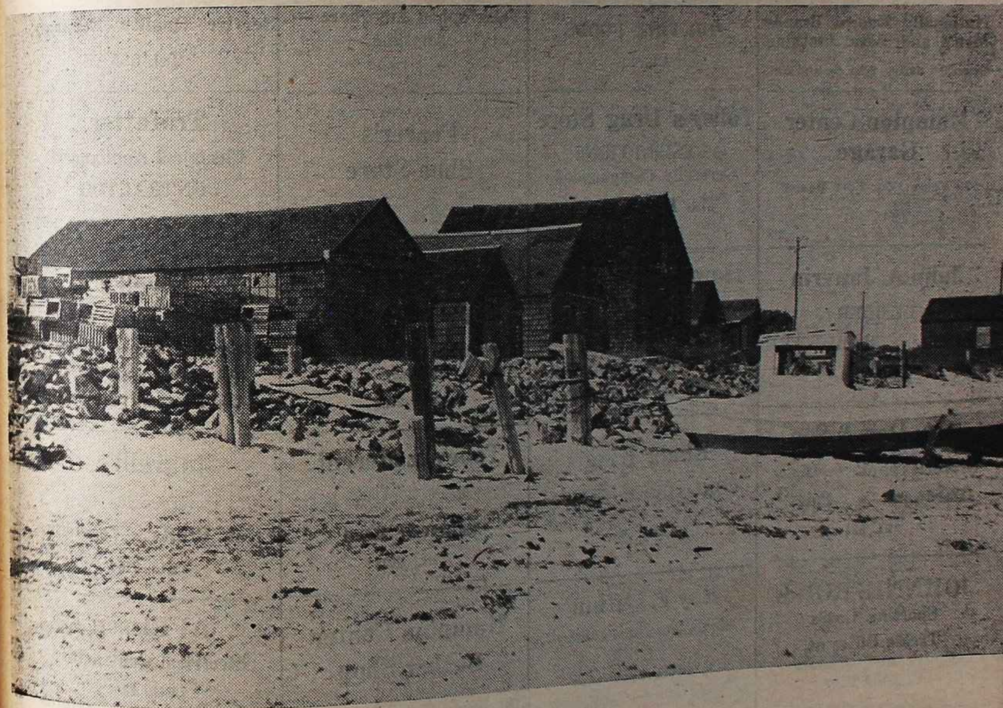
FISH HOUSES AT NORTH BEACH
